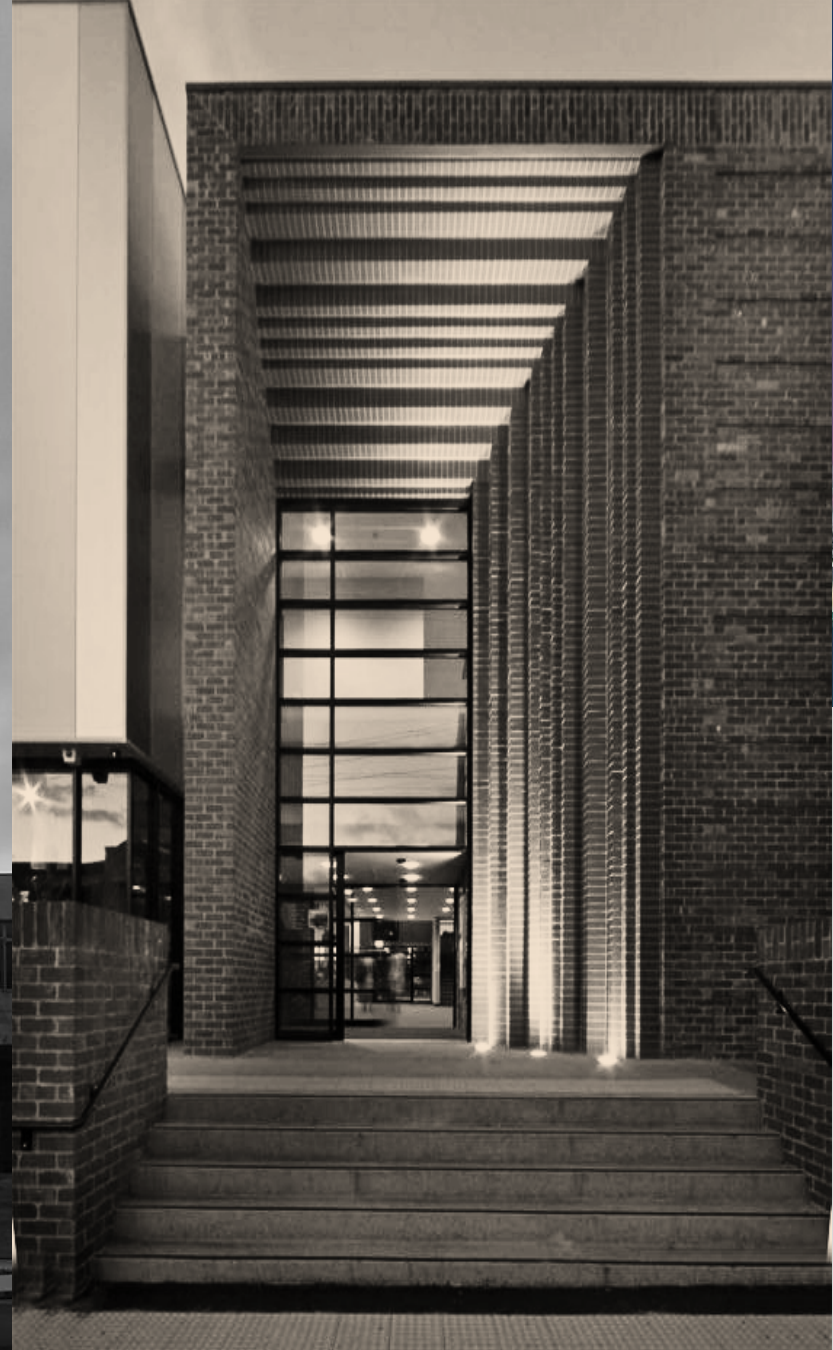
North Melbourne Reserve, Williams Ross Architects
